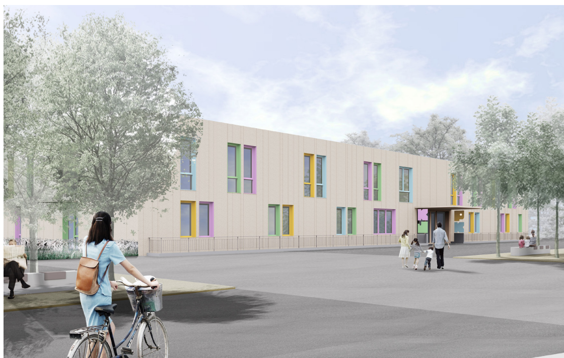
'KJPK' CHILDREN'S PSYCHIATRIC CENTER. The exterior walls are regulated by a strong orthogonal arrangement and are intentionally generic. They are finished with fiber cement panels. Once inside the building, the voids dominate the composition.
