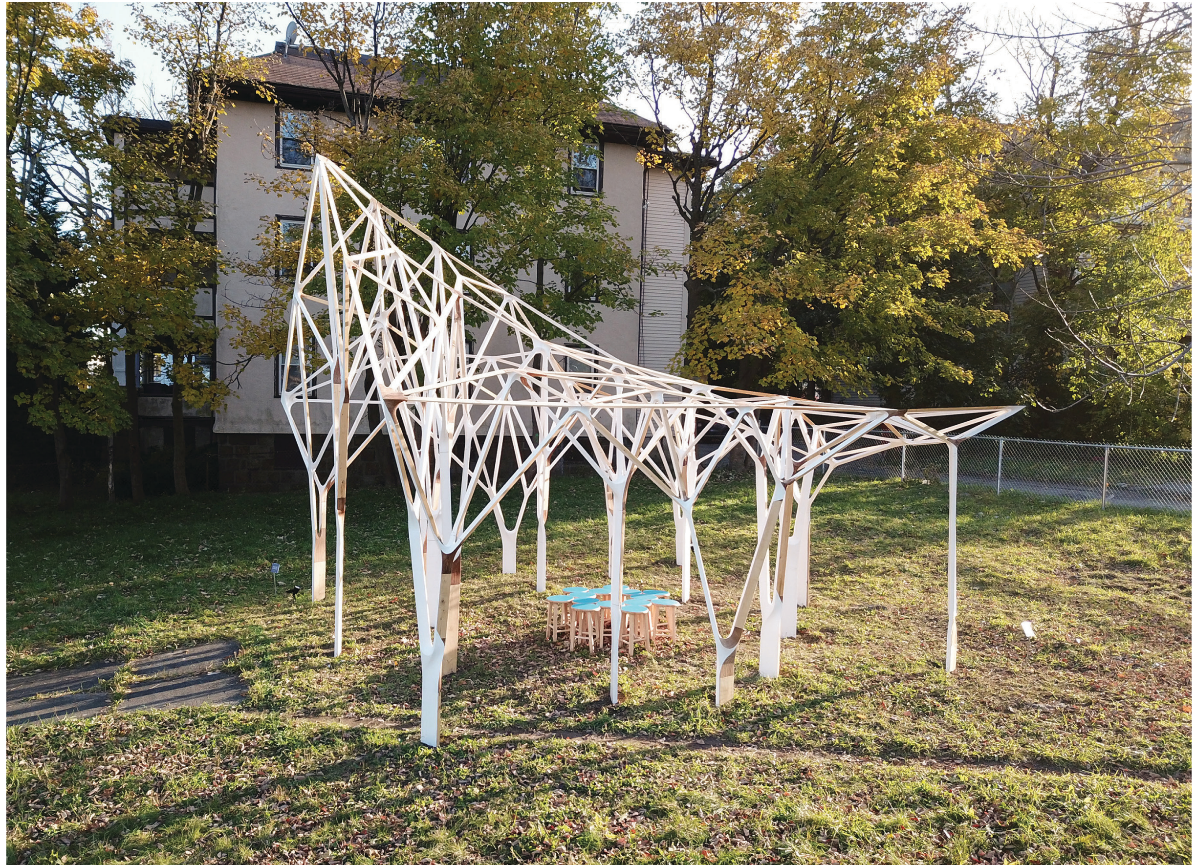
Lost House. A structure that creates new public space out of a vacant lot in a vibrant residential neighborhood. Conventional wood framing members are joined with custom CNC-milled nodes to create branching structures and a global form that is like a house, and yet not a house. Self-structured sub-assemblies are joined together in the customized Kagome truss.
